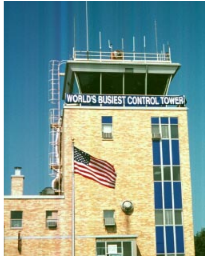
The FAA tower at Oshkosh.
