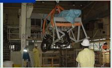
NASA used the 100-kilowatt Mock-Up Reactor - a near duplicate to the main reactor but having a very low-level radioactive environment - for training exercises leading to segmentation of the main 60-megawatt reactor. Further disassembly of the Mock-Up Reactor, shown right, was completed in early 2004.
