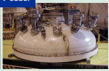
The reactor pressure vessel head was removed and eventually cut or segmented, into 3 pieces for packaging, shipping and disposal.
