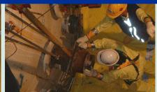
Horizontal Beam Tubes - metal pipes running through the vessel wall up to the core box - contained higher amounts of radioactivity and were the first components removed using specially made remote tools to withdraw, cut and lift the tubes out of quadrant D and into a shielded waste container.
