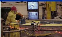
Cameras in the reactor vessel provided real-time video of internals removal. An operator, shown left, helps guide the worker, shown right. The worker stood behind steel barriers and reached into the vessel using long-handled tools - keeping him a safe distance and minimizing the potential radiation dose.
