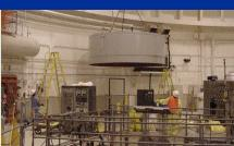
One of three 20-ton metal shrapnel shields covering the reactor lid was lifted off to cut a hole in the middle, then replaced to serve as an extra barrier - protecting workers from radiation exposure as they removed components from the reactor vessel.
