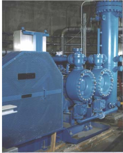
High Pressure Piston Diaphragm Pump used to convey 60% solid slurry one mile to BSA
