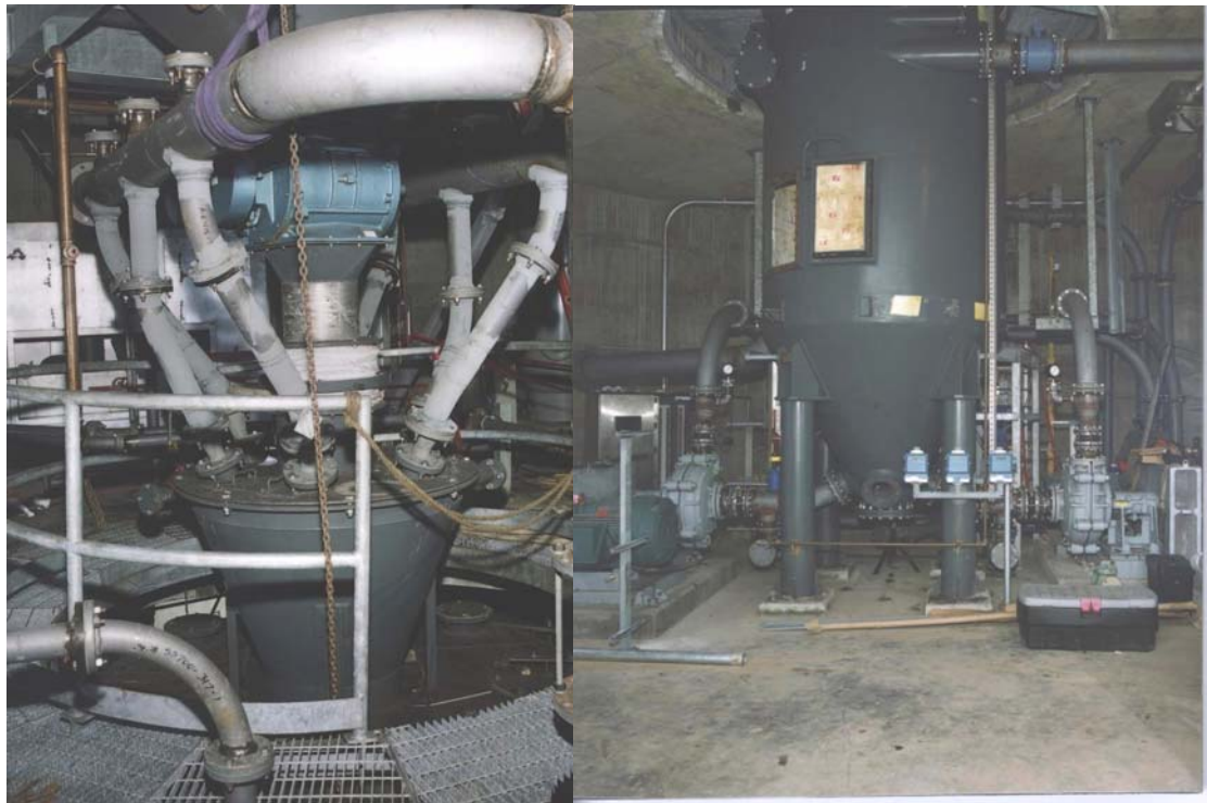
Left Photo - Fly Ash mix tank top showing inlet rotary vane feeder and premixer. Right Photo – Bed Ash mix tank showing mixing pumps.
