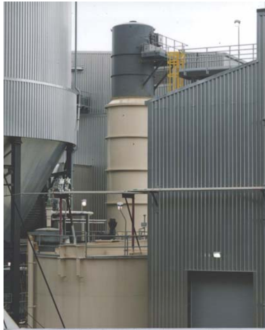
Recycle Storage Silo (tan) with integral Filter/Separator on top (gray)
