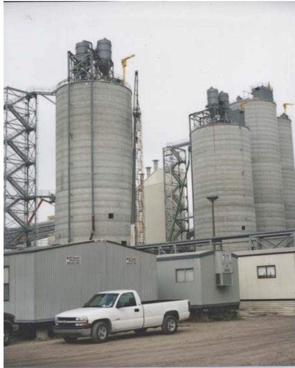
Ash storage silos, two fly ash silos on the left, two bed ash silos on the right
