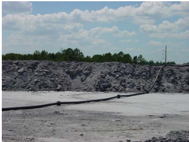
Poly pipe routed over dike on recently placed high density slurry.
