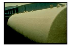
This is a picture of a **tank** made of steel clad with a thick layer of noncorrodible material.
