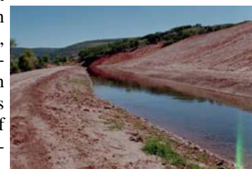
Repaired ditch prior to reseeding
