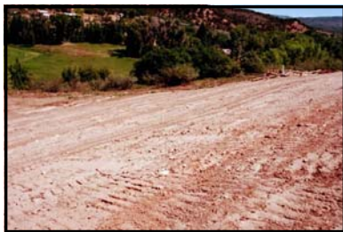
Area below ditch before
