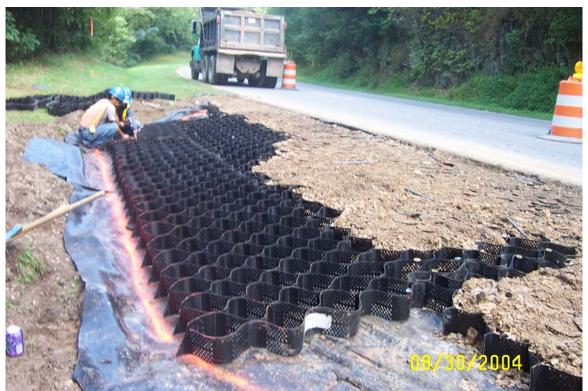
Figure 2. Geoweb placement and backfill with engineered aggregate-topsoil.
