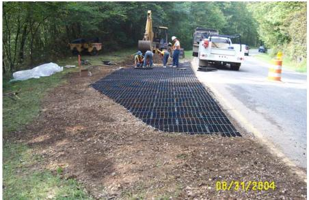
Figure 4. Geoblock installed and cut to fit the pull-off at PA #3.
