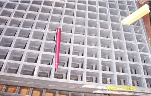
Figure 7. The fiberglass grates for this project were one-inch deep and were delivered in  $4' \ge 10'$  sheets. The panels for this project were pre-cut to the shape of the parking areas.
