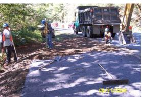
d. Aggregate-topsoil cover for turf establishment.
