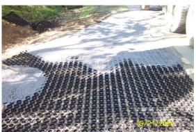
c. Backfill consisting of AASHTO #89 stone.
