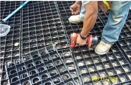
Figure 3. Porous cellular block panels (geoblocks) placed in pull-offs #3 and #4.
