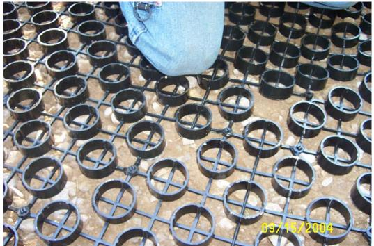
Figure 5. The ring and grid is shown here after being snapped together at the joints.
