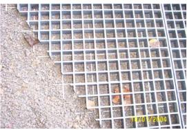
b. Grate placed on weld wire fabric and #89 stone.
