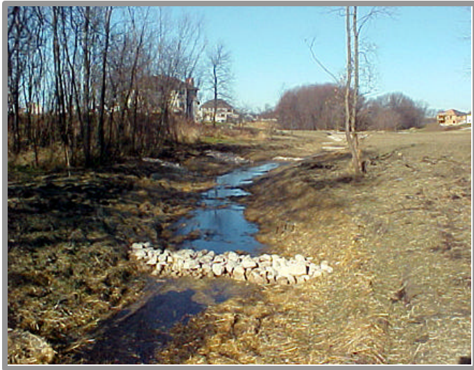
Figure 7. Erosion control matting and a rock check dam combine to reduce stream channel erosion and enhance storm water infiltration in developed headwater areas.
