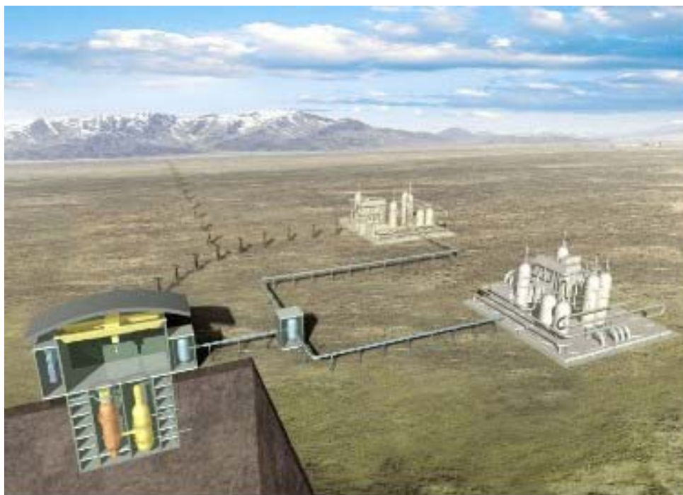
Figure 1. An artist's conception of a direct cycle very high temperature gas cooled reactor and associated hydrogen production plants.
