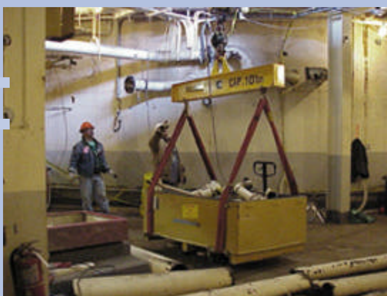
Workers load a box with fixed equipment.
