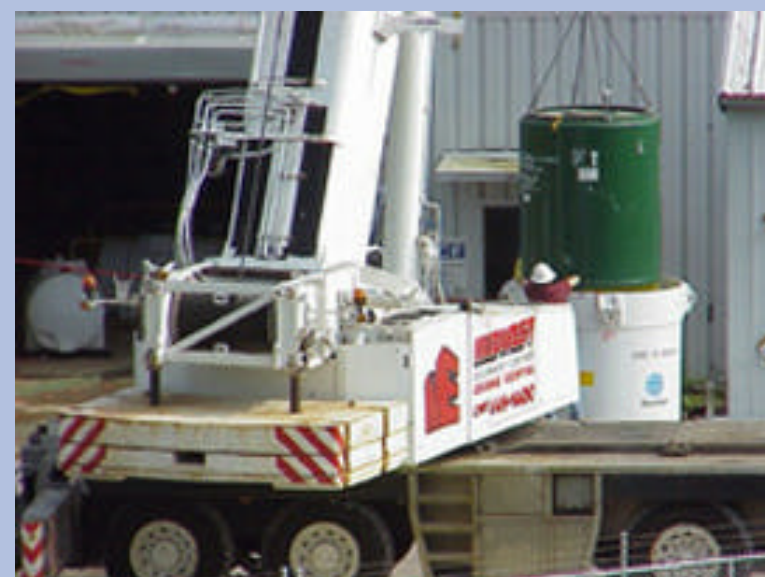
A steel liner containing segmented reactor internals is placed in a shipping cask (left). The cask sits on a flatbed truck as it leaves Plum Brook Station for the Barnwell licensed disposal facility in South Carolina.
