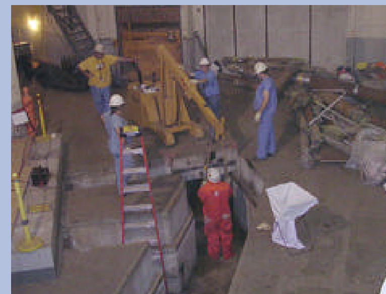
At the (-25) foot level of the Reactor Building, workers cut pipes down to the bare walls, leaving only stubs (left). They are also using this area to stage the packaging of cut pipes moved from other Reactor Facility buildings (right).
