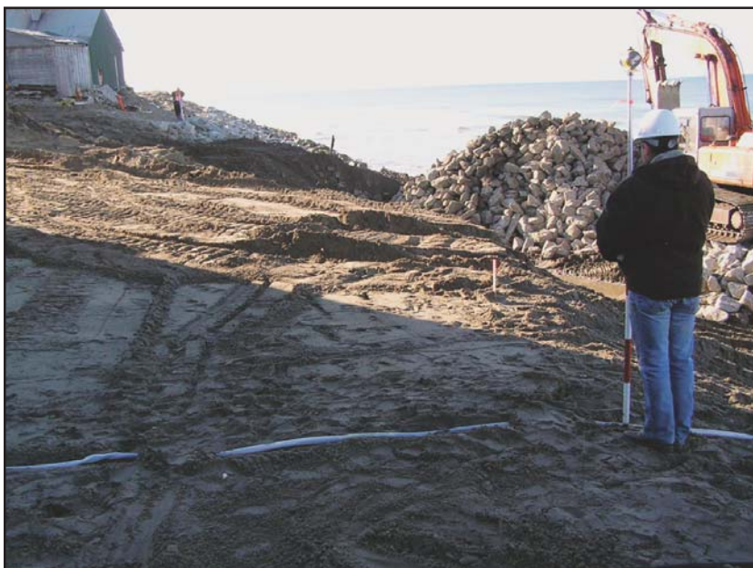
Installation of a thermistor during the Shishmaref shoreline protection project.
