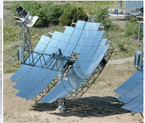
The six-dish Model Power Plant at SNL facilitates SES dish/engine R&D, including system development and reliability improvement.
