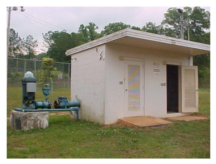
Figure 1: Grant Street Well – Note missing section of pipe.
