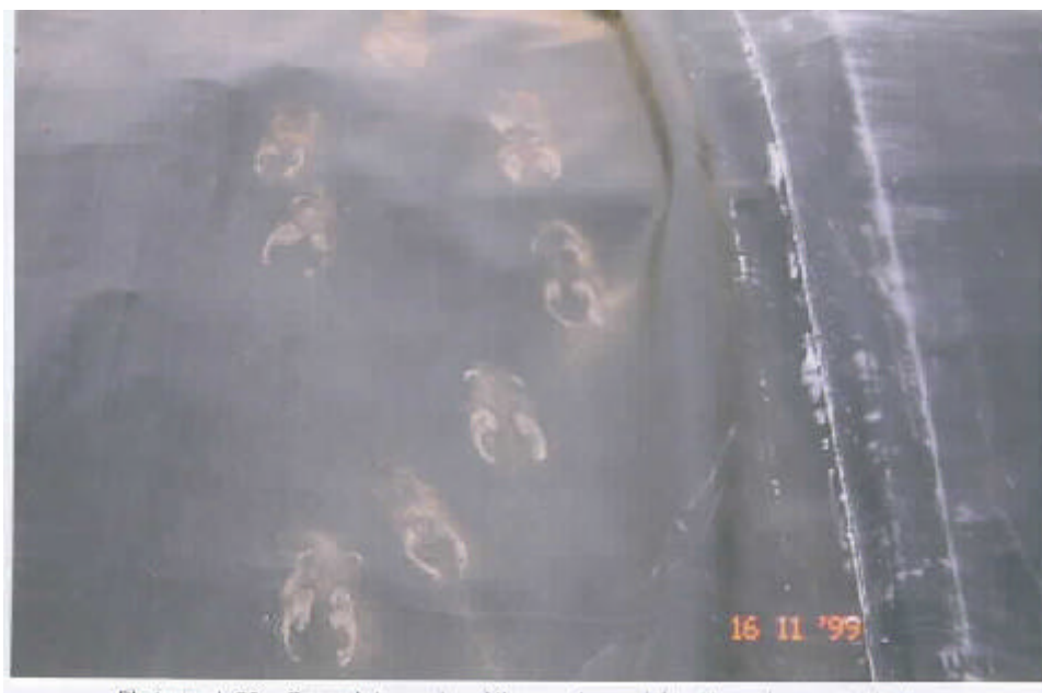
Photograph 20.—Several deer entered the canal overnight with no damage to the liner. Also note the close-up of the vulcanized factory seam on the right.
