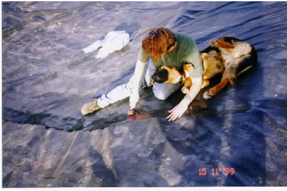
Photograph 14.—The tape is then rolled to seal the seam and remove any wrinkles.
