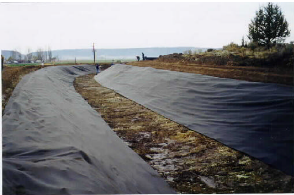
Photograph 4.—Geotextile is unrolled along the canal bank and pulled into position
