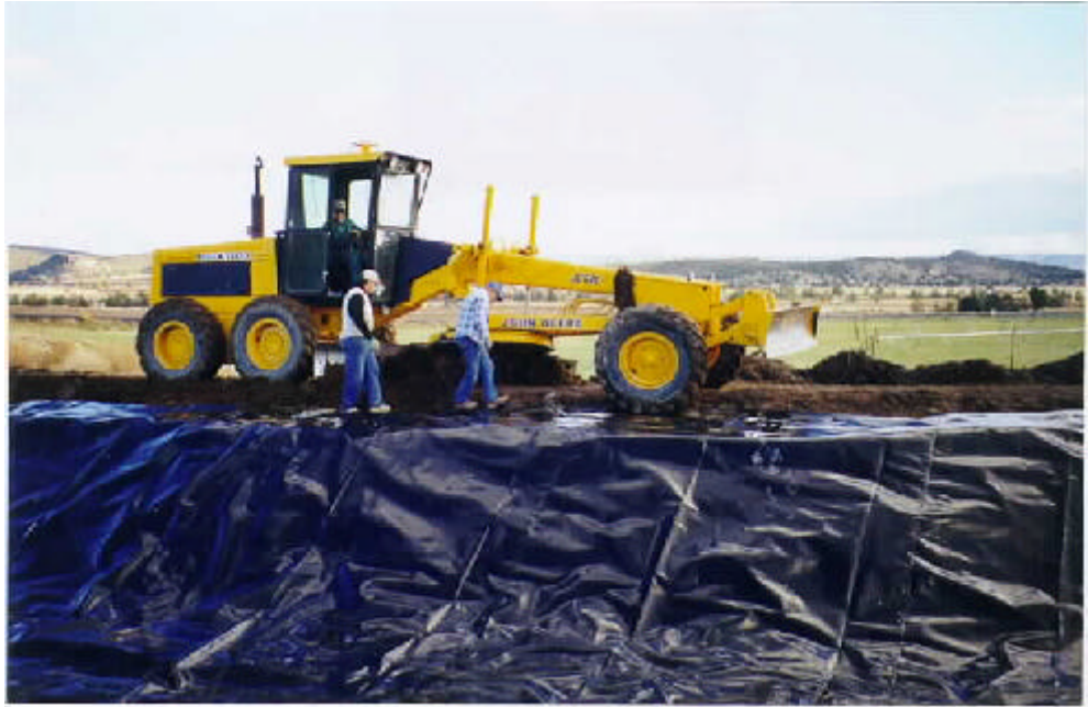
Photograph 17.—Grader backfills the V-notch anchor trench.
