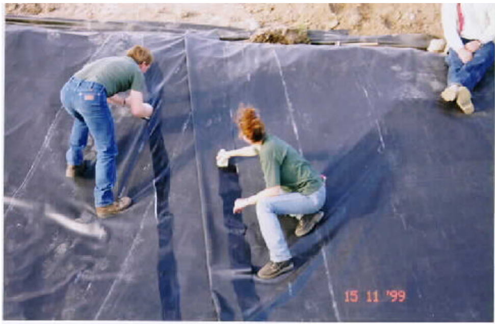
Photograph 10.—Adjacent panels are shingled downstream, and primed on both surfaces.
