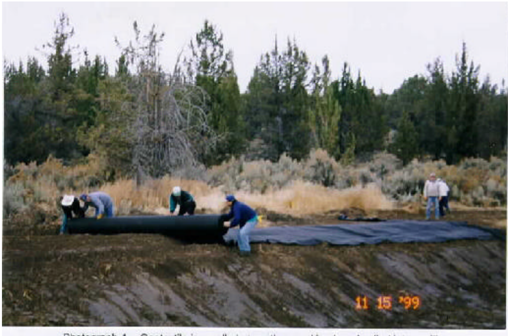
Photograph 5.—Geotextile covering the sideslopes; Manufacturer did not require geotextile in the invert.
