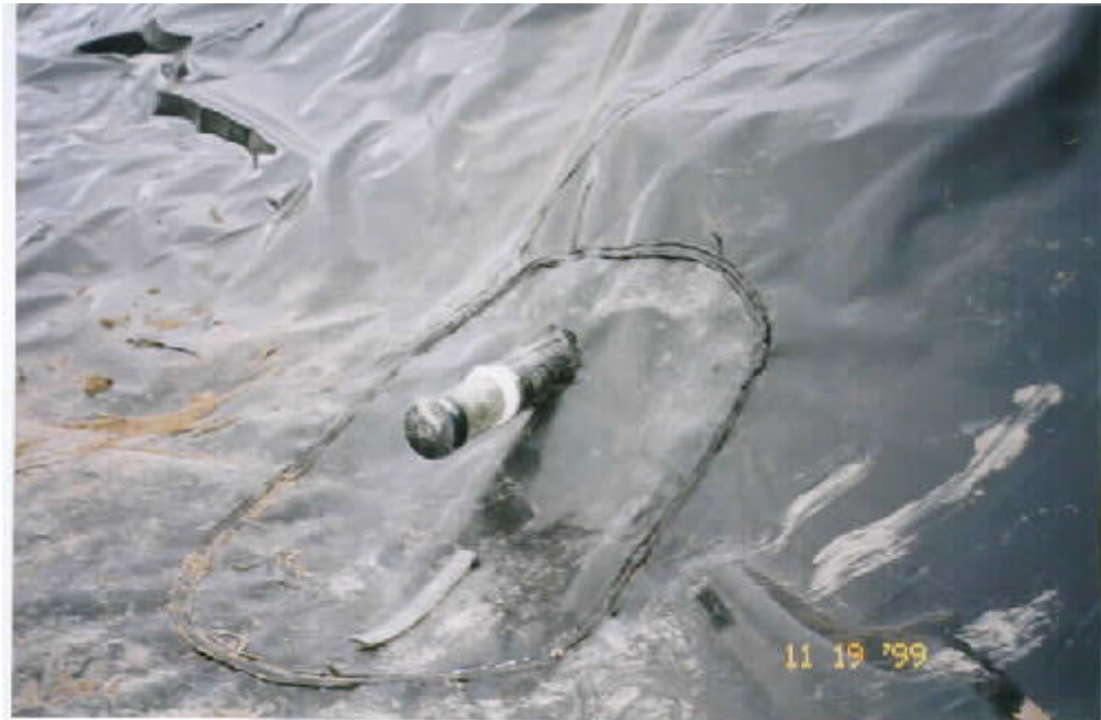
Photograph 15.—Completed pipe boot around 4-inch pipe penetration.
