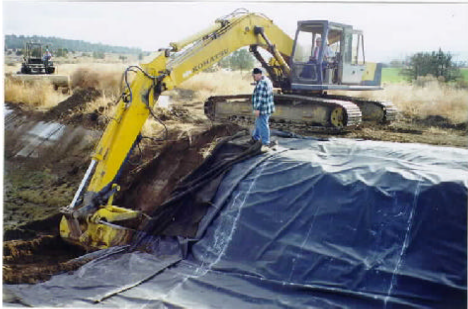
Photograph 17.—Trackhoe excavates cut-off trench at the upstream transition.
