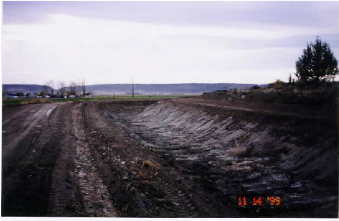
Photograph 1.—The Ochoco Irrigation District prepared the subgrade by removing vegetation, restoring the 1½:1 sideslopes, and cutting the V-notch anchor trench.
