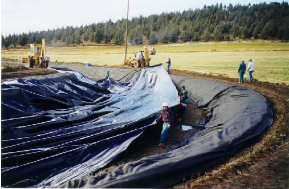
Photograph 7.—Larger panes (up to 250 feet long) are unfolded by two backhoes operating on opposite banks.
