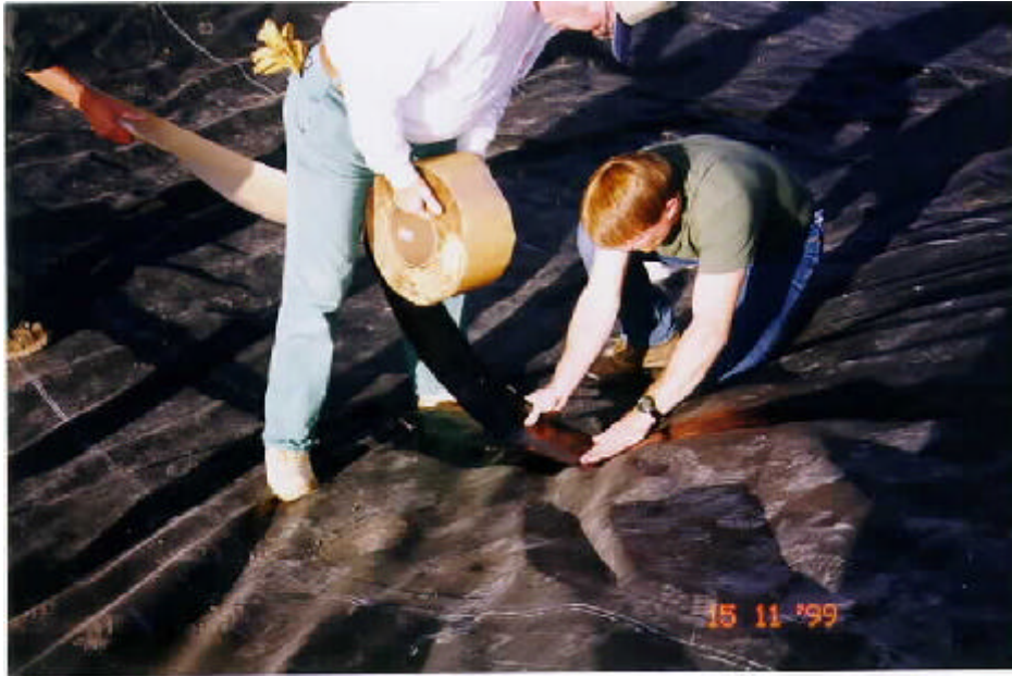
Photograph 13.—The top surface of the seam is then primed and covered with 6-inch-wide EPDM tape.
