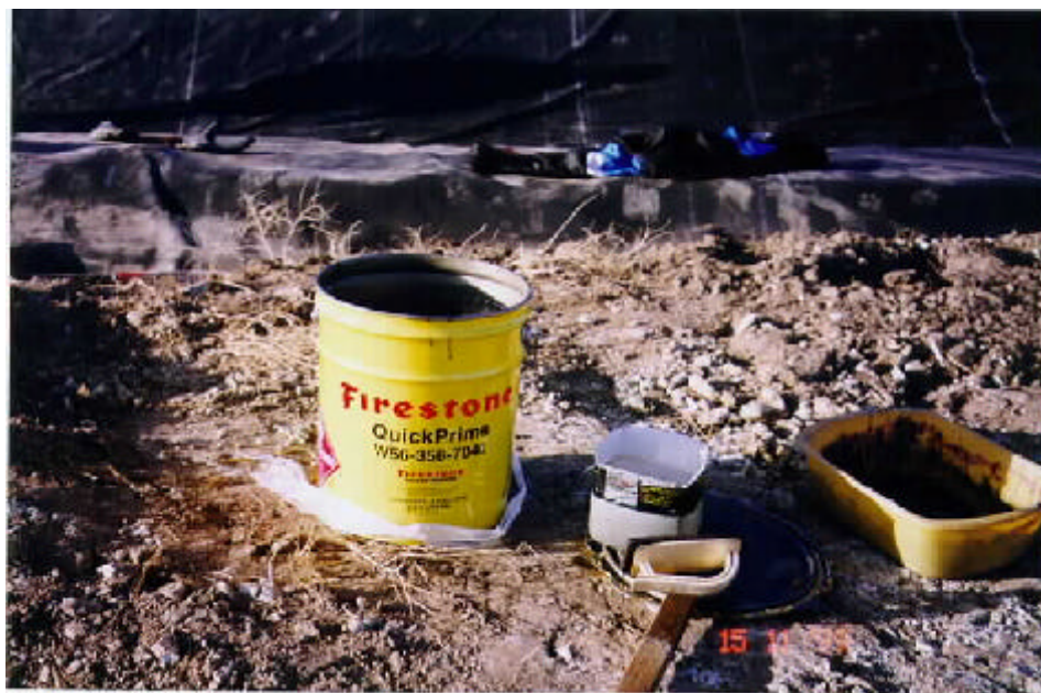
Photograph 11.—Firestone “Quick-Prime” acts as cleaner, primer, and adhesive.
