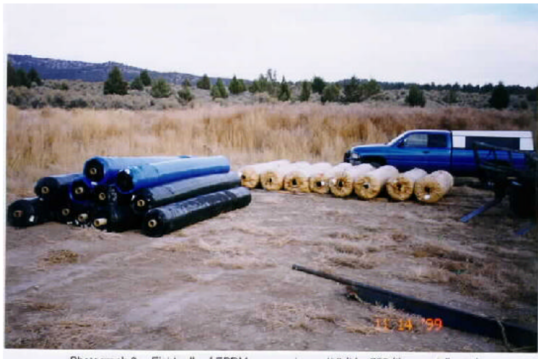
Photograph 2.—Eight rolls of EPDM geomembrane (50-ft by 200-ft) were delivered to the jobsite; Rolls of geotextile cushion (foreground) measure 15-ft by 300-ft
