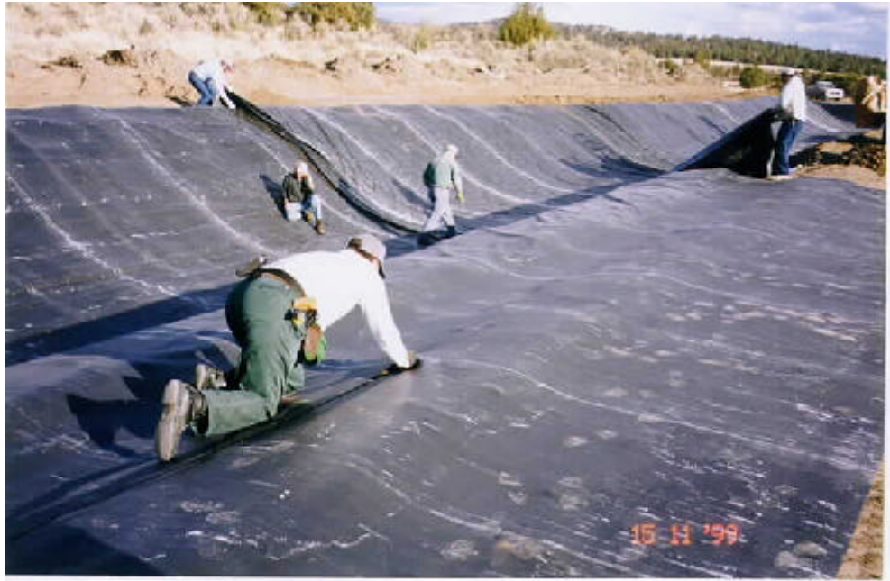
Photograph 9.—After final positioning, excess material is trimmed and discarded. Note that the factory seams run across the canal (perpendicular to flow).
