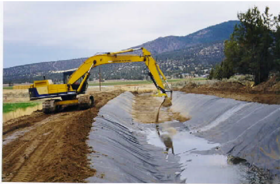
Photograph 21.—Trackhoe places 4 to 6 inches of soil cover in the invert on the downstream half of the test section. Upstream half is left entirely exposed. Note the rain water that has collected in the invert overnight.
