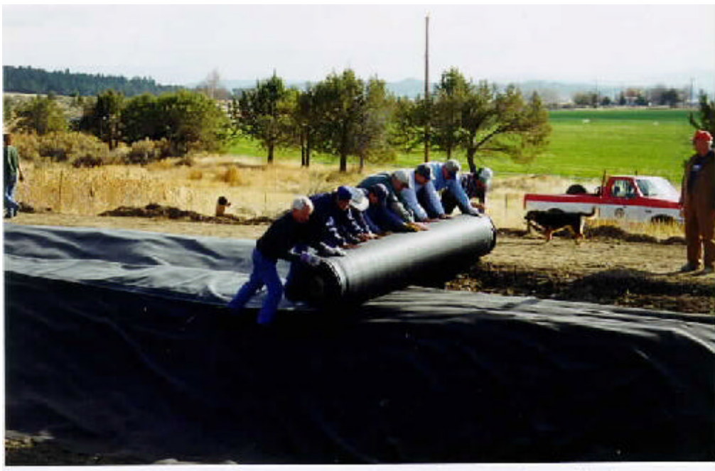
Photograph 6.—Crew unrolls the EPDM geomembrane along the canal bank.
