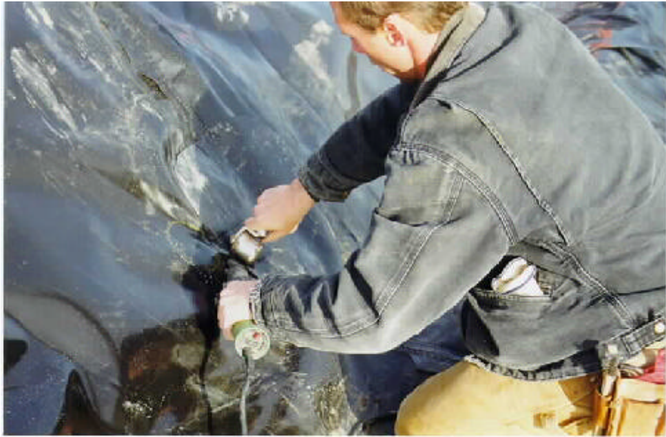
Photograph 11.—Welding technician patches the liner with hot-air welder.
