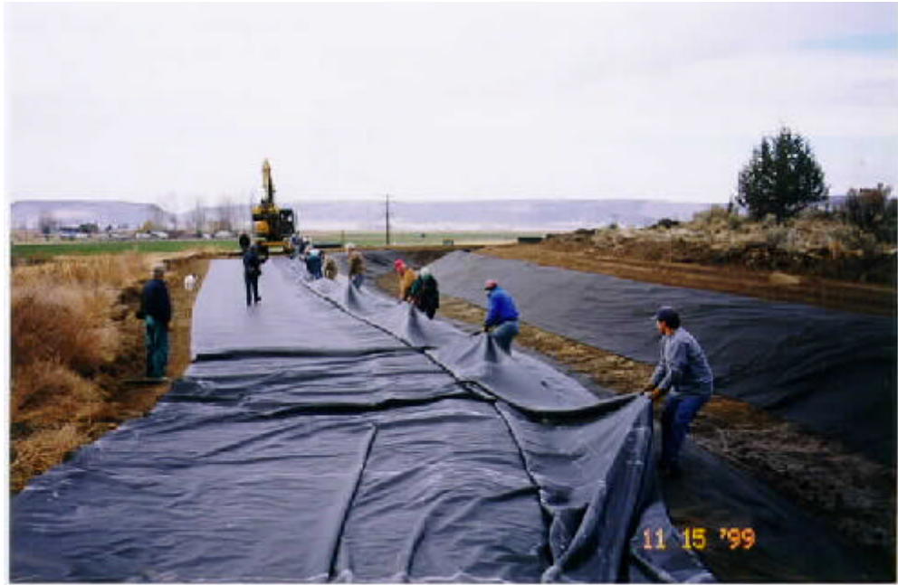
Photograph 7.—Crew unfolds the EPDM membrane into the canal prism.
