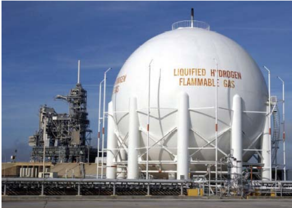
Figure 32. Complex 39 Liquid-Hydrogen Storage Facility
