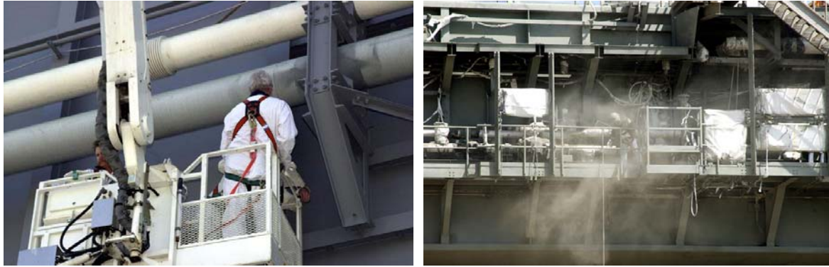
Figure 27. MLP Propellant Line Repair and Routine Sandblasting
