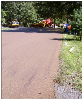
Richmond National Battlefield Park Rustic Pavement Test Strip — Clockwise: Gravel Aggregates Used, Paving With 9.5mm Tan Gravel, Paving with 12.5mm Brown Gravel, Synthetic Binder
