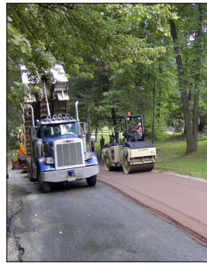
Paving Operations — 9.5 mm Superpave Field Test, Rock Creek Park, Washington, DC.
