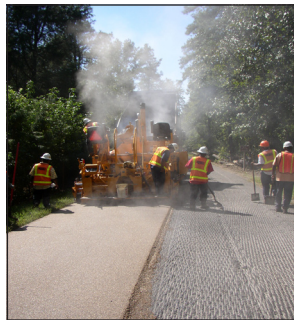
Richmond National Battlefield Park Rustic Pavement Test Strip — Clockwise: Gravel Aggregates Used, Paving With 9.5mm Tan Gravel, Paving with 12.5mm Brown Gravel, Synthetic Binder
