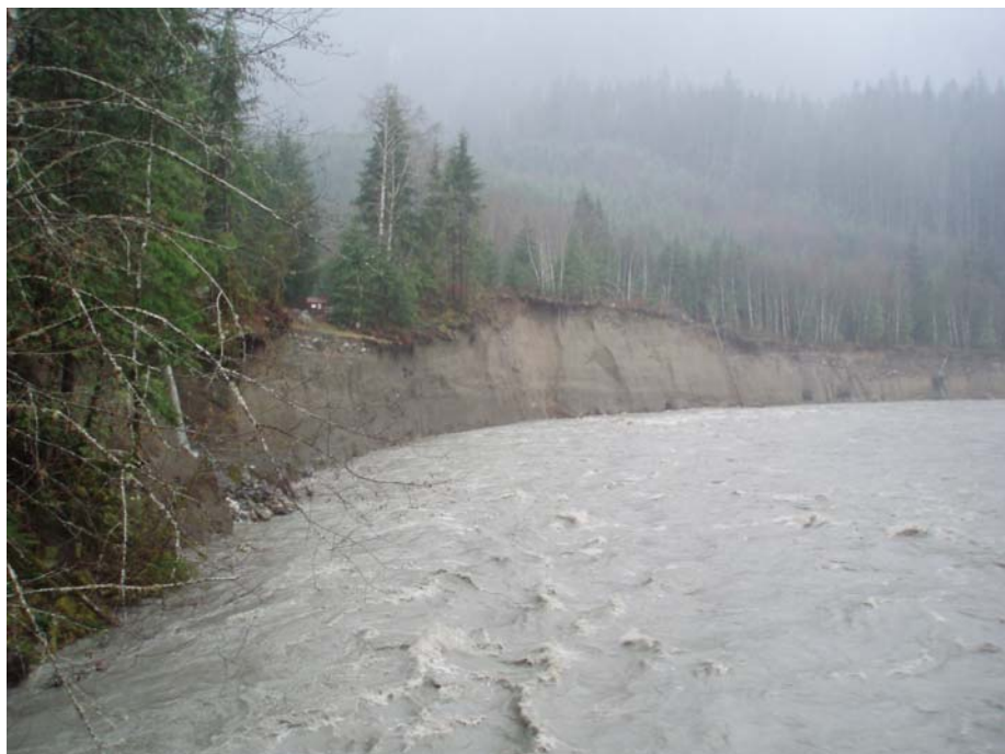
Washout site on December 3, 2007 during high flow (looking downriver from Blue Bridge).
