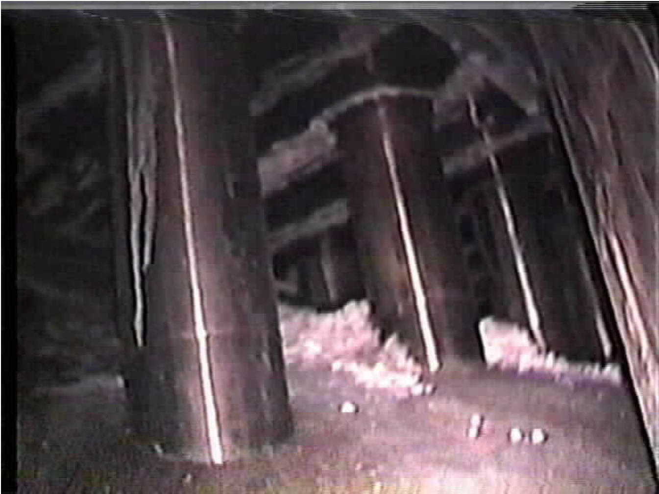
Figure 33. North Side of Reactor Vessel Head (10RFO)
