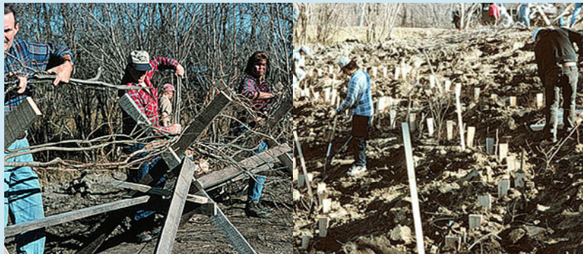
The Natural Resources Conservation Service demonstrated the implementation of several bioengineering techniques during a workshop (left). Willows were planted along the restoration site to provide long-term stability (right).
