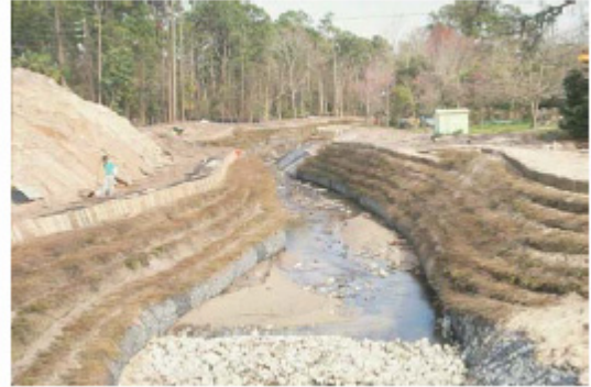
Figure 3.31 VRSS Structure After Construction (Source: Sotir and Fischenich, 2003)
