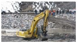
2 pm: Removing material to begin the breach of the spillway coffer dam and divert the Clark Fork and Blackfoot Rivers into the new channel
