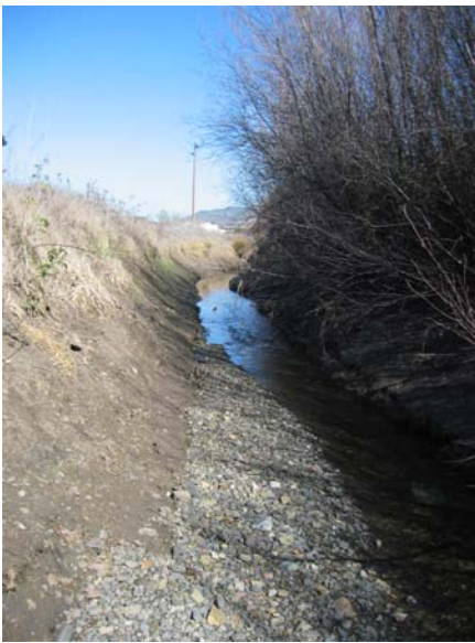
Figure 9. View of MID canal from the canal near the South Fork Larson diversion structure. This is the portion of the canal that would function as restored stream channel as described in the Preferred Alternative.
