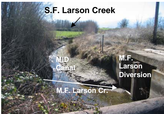
Figure 6. The MID diversion at Middle Fork Larson Creek. Riparian vegetation adjacent to South Fork Larson Creek is visible in the background. Flashboards are not in place.
