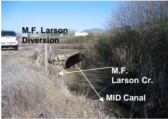
Figure 5. The MID diversion at Middle Fork Larson Creek and the MID canal.
