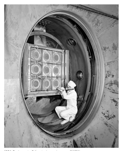
1964: Engineer at a 9 thruster ion engine array. (NASA)
