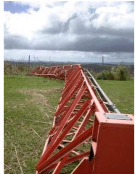
This antenna was toppled by high winds.
