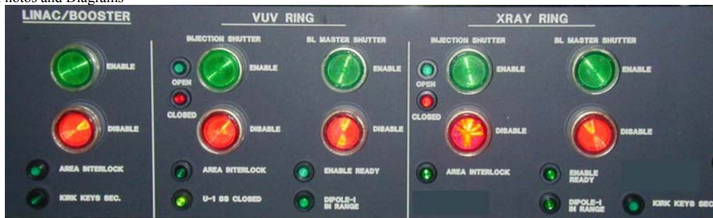
Figure 1: Injection Control Panel (located at Operator's Console)
