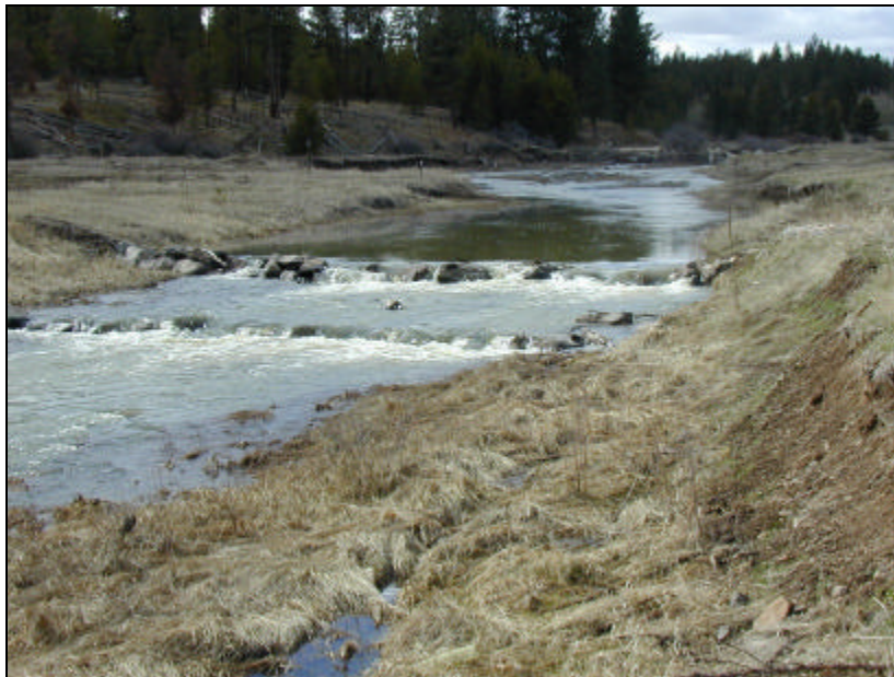
Channelized McCoy Creek downstream from diversion. Rock structures in middle-ground installed to trap sediment and aggrade stream channel for future restoration.
