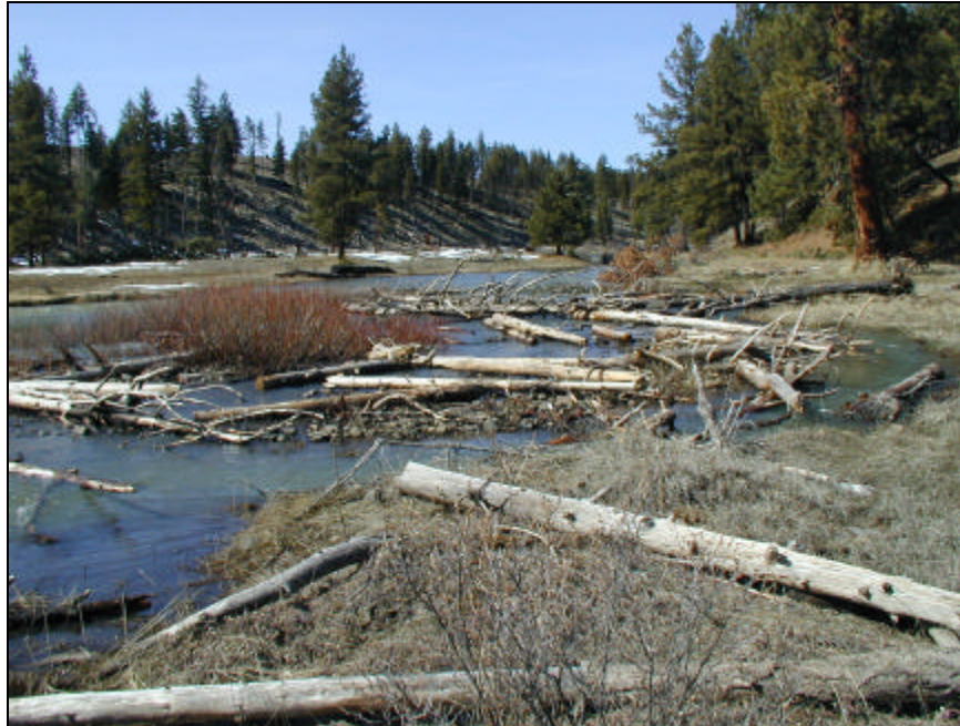
Large woody debris installed to stabilize gravel bar and provide cover and backwater habitat during spring flow periods.
