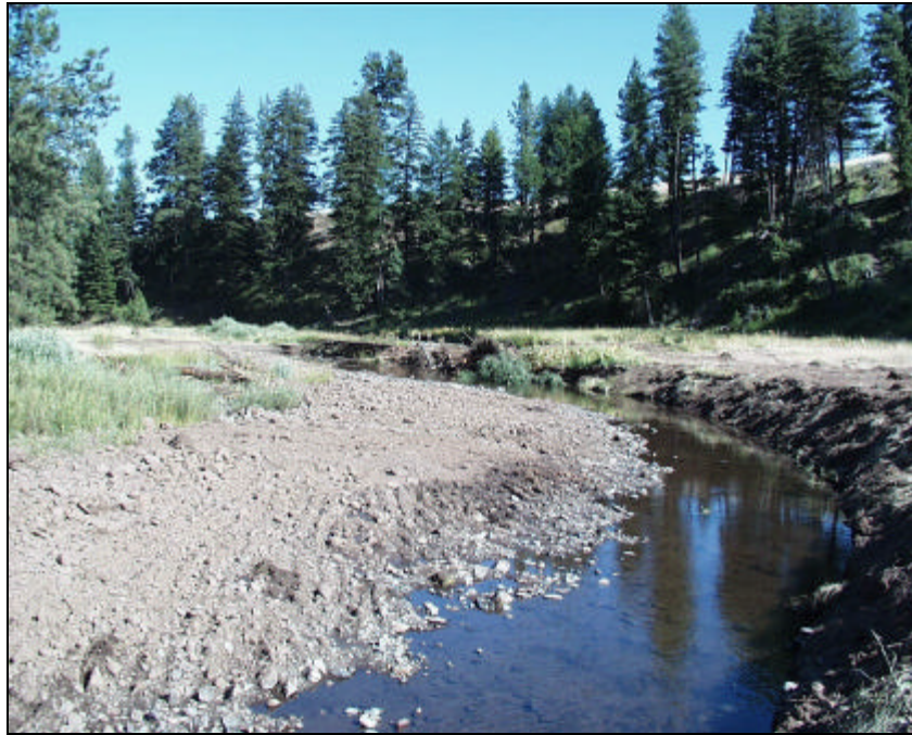
Outside stream channel meander construction to decrease stream gradient, increase channel length, and restore fluvial processes
