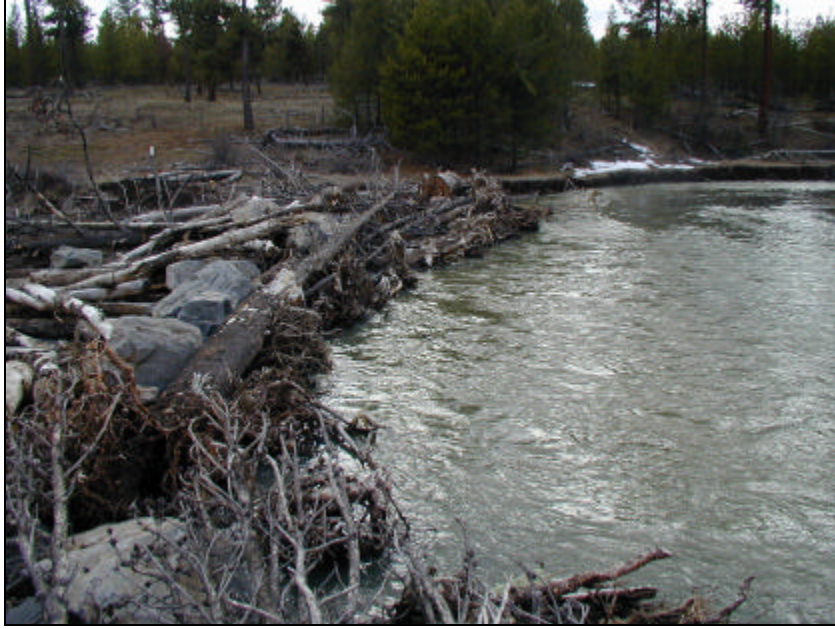
McCoy Creek 1997-98 Diversion Structure
