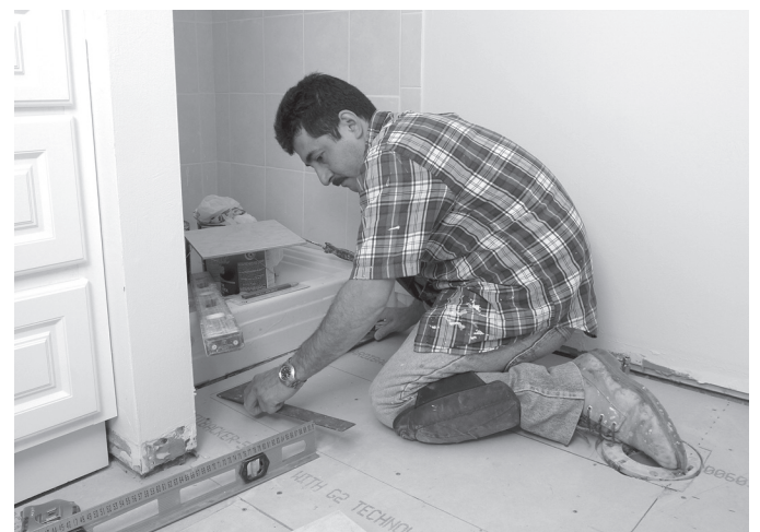
Prior to installing tile, tilers use measuring devices and levels to ensure that the tile is placed in a consistent manner.
