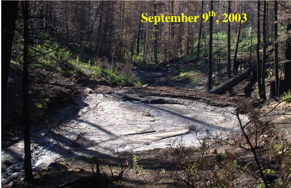
Figure 28 – A check dam full of mud and debris constructed in the upper reaches of Basin MR-61 above Lemon Dam (photo from FWCD, 2003).
