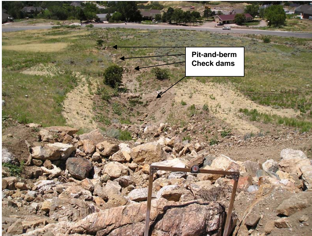
Figure 6 – Excavated pit and berm style check dams in Farmington, Utah.
