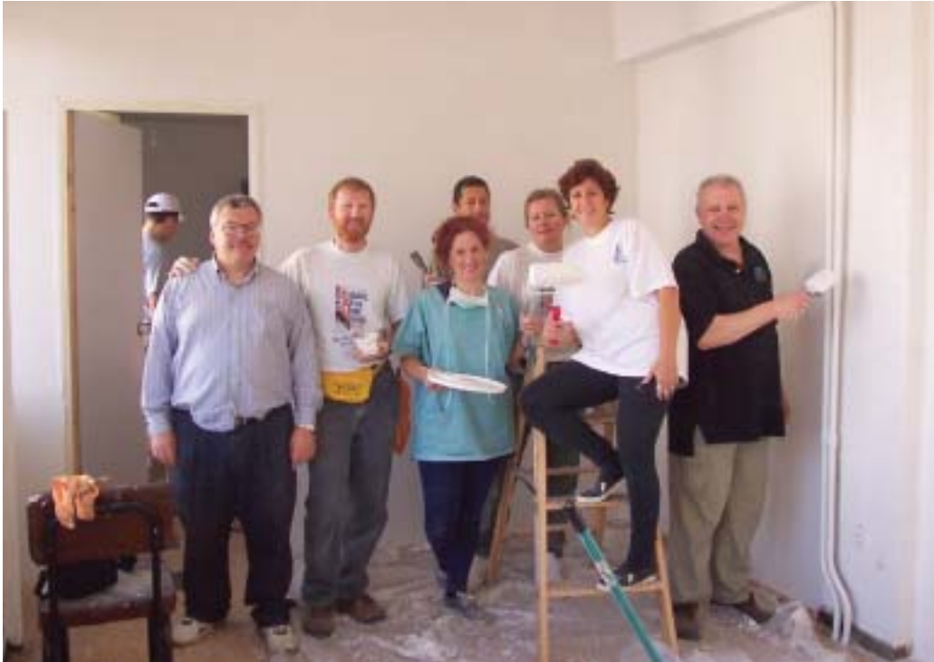
Members of the Community Service Network refurbish a community shelter in Athens. Below: Vassilios Tsiboukis from the Public Diplomacy Information Resource Center, left, and Debi Guido-O'Grady, Olympic Information Officer, help open a new American Corner in a Xanthi library.
