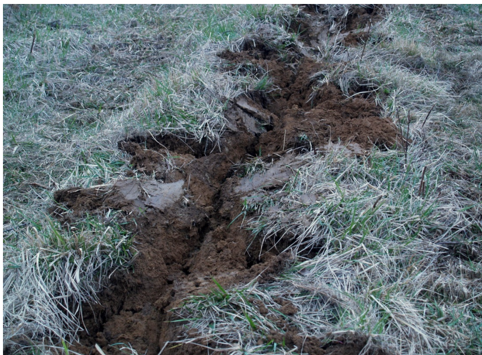
Figure 3. Soil shown ripped 1.5 ft. with ripper attachment on a bulldozer.
