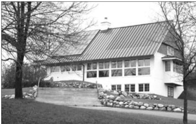
The recently completed “Nature House” at the Leslie Science Center in Ann Arbor, MI, is an environmental learning center that combines PV with other solar technologies. Features include a First Solar 2-kW solar-electric array composed of CdTe thin-film modules; solar thermal panels for heating water; windows designed for direct-gain sunlight in winter; and an 8-inch Trombe wall for heat storage. Energy-efficient features include compact fluorescent lighting and appliances.
