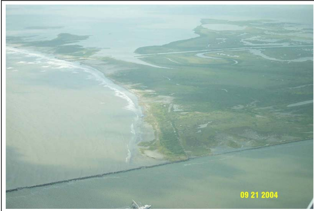
Figure 21. September 2004 aerial image depicting shoreline transgressions in the beach fill and project areas at the West Belle Pass Headland Restoration (TE-23) project.
