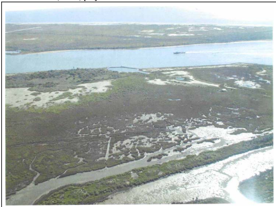
Figure 12. February 2003 aerial view of severe marsh tracks located just east of the Louisiana Intrastate Gas Pipeline Canal in the vicinity of the closure 1 marsh creation area at the West Belle Pass Headland Restoration (TE-23) project.
