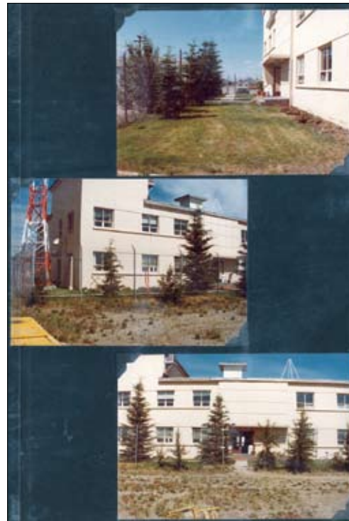
Above: The old FAA building- still home of the Galena (winter), Tanana, Upper Yukon, and Military Zones on the second floor, and on the first floor the Branch of Technical Systems.
