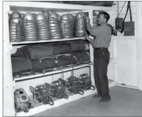
Firefighter gear stored at the warehouse.
