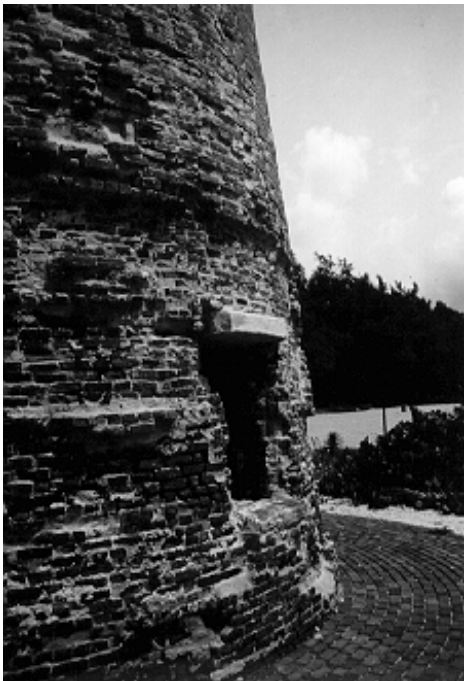
Figure 26. View of the lower tower window; note the depth of the brick deterioration at the window openings. The face of the protruding granite lintel above the window opening represents the face of the original wall.
