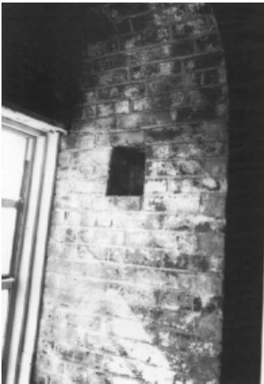
Figure 13. Vent hole located in the window well of a brick lighthouse.
