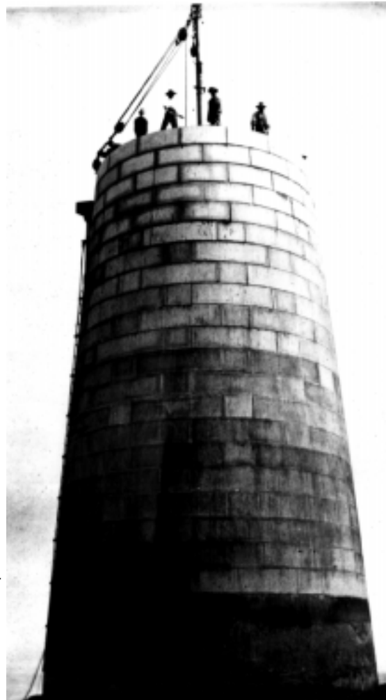
Figure 31. Work on Minots Ledge Lighthouse as it progressed just above the entrance level which is visible on the left. The tower below this level was essentially solid.
