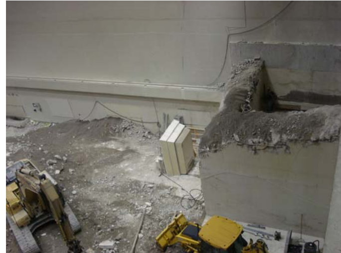
Hot cell 6' thick wall cut
