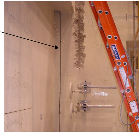
Hot cell 6' thick wall cut
