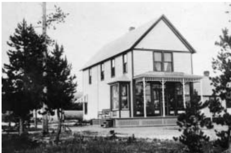
The Klammer store prior to Reamer’s remodeling.
