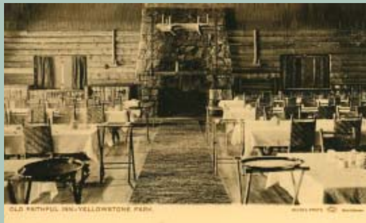
The dining room chimney collapsed and the fireplace cracked in the quake.
