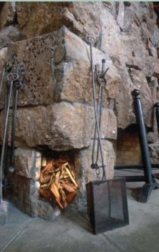
To increase seismic stability, the four corner "kindling" fireplaces will be filled in with concrete piers.
