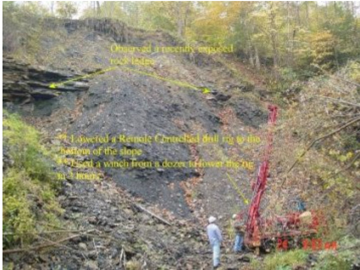
Figure 4. Slope toe retaining wall borings drilling operation
