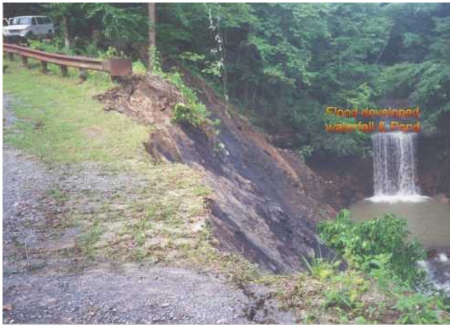
Figure 3. Flood reshaped waterfall located near upstream end of landslide
