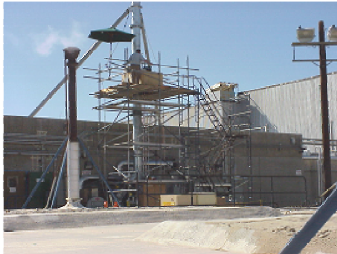
Figure 2.1. Stack and Temporary Scaffold
