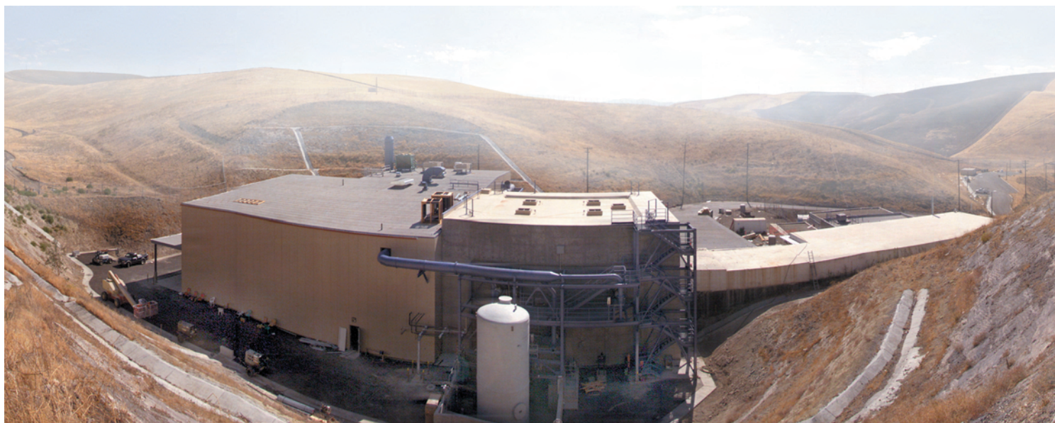
At Livermore's Site 300, Bunker 801 became the Contained Firing Facility when the bunker's open-air firing table was enclosed in 2000. The enclosure reduces emissions to the environment and minimizes the generation of hazardous waste, noise, and blast pressures. Construction of the firing chamber required 3,200 cubic meters of concrete and more than 2,000 metric tons of steel reinforcement. Equipment and diagnostic upgrades at the facility have greatly improved the quality of data gathered from hydrodynamic tests of mock weapon primaries.
