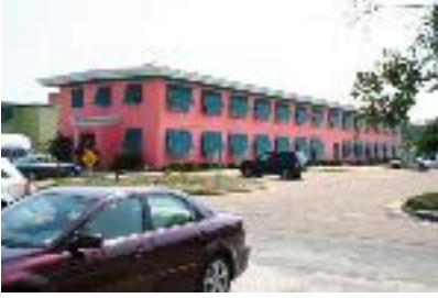
Hurricane shutters protect a Sea Lab building.
