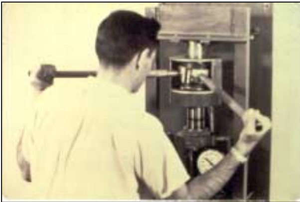
Figure 1. Texas Gyrotory Press
