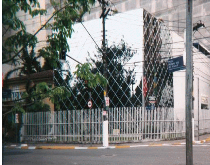
Figure 5: The US&FCS Post and Commercial Center in São Paulo
