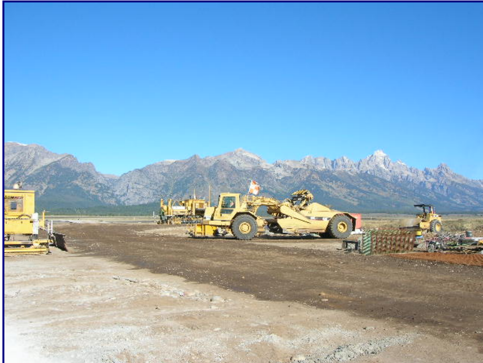
Commercial Service Apron Expansion, Jackson, WY
