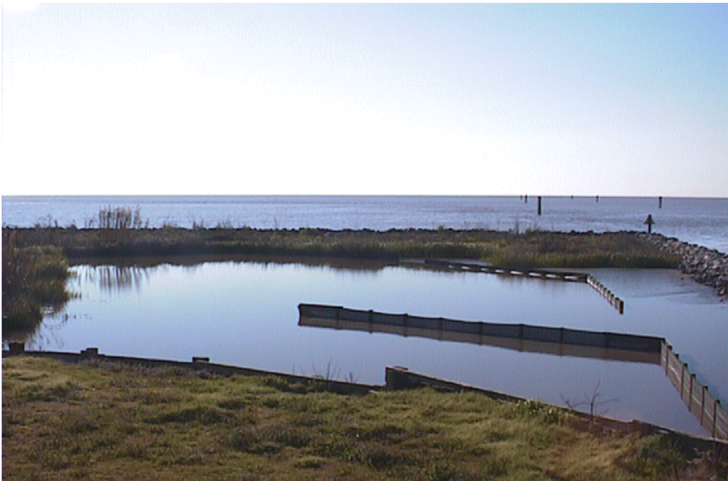
Figure 12. Boston Canal/Vermilion Bay Shoreline Protection (T/V-09) photographs: (A) sediment deposition, December 1994; (B) vegetation behind rock breakwater; February 1998.
