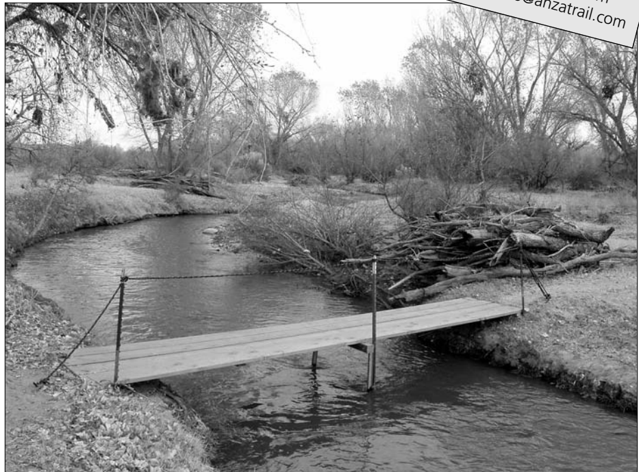
Footbridge across the Santa Cruz River is designed to swing out of the way during monsoon floods without washing away. Photo: ATCA
