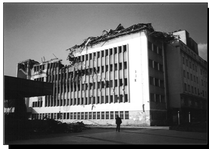
Result of NATO bomb on post office used by Yugoslav forces in Pristina, Kosovo Source: GAO.
