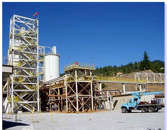
Photo 4: The lime neutralization/high-density sludge acid mine drainage treatment facility at Minnesota Flats.
