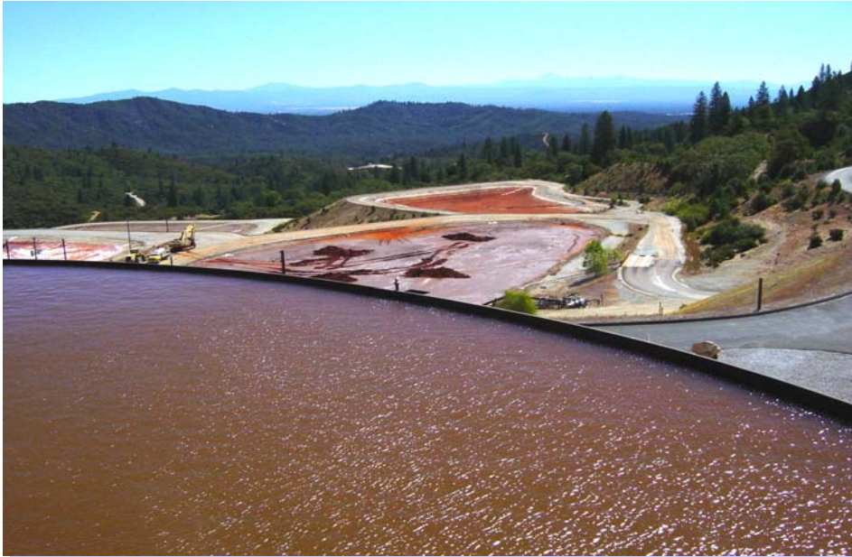
Photo 7: The sludge conditioning tank at Iron Mountain Mine is one of the largest in the world. The sludge is periodically transferred to the drying beds visible behind the tank before being placed in a disposal cell on the site.
