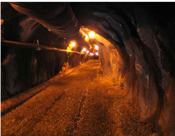
Photo 3: The view looking into the refurbished Richmond adit. The pipe used to convey acid mine drainage out of the mine is visible on the tunnel floor at left.
