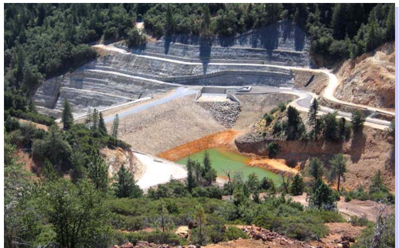
Photo 9: The recently completed Slickrock Creek Dam captures acid mine drainage escaping from fractured bedrock and buried mine portals along the south side of Iron Mountain. The water in the reservoir is transported by pipeline to the treatment plant at Minnesota Flats.
