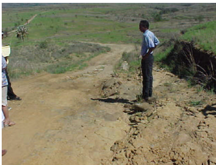
Road Rehabilitation in Isalo, funded by FCV Japon
