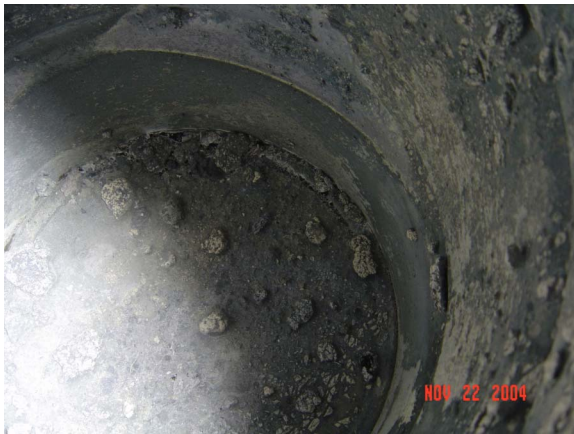
Figure 14. ANL#1174 prior to treatment
