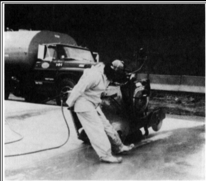
Figure 6. Sawing of concrete pavement containing crystalline silica during highway construction.
