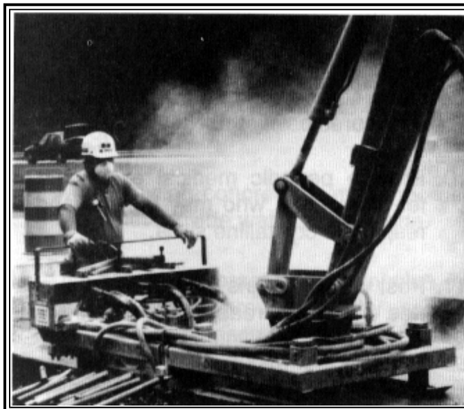
Figure 4. Drilling of concrete pavement containing crystalline silica during interstate highway repair.
