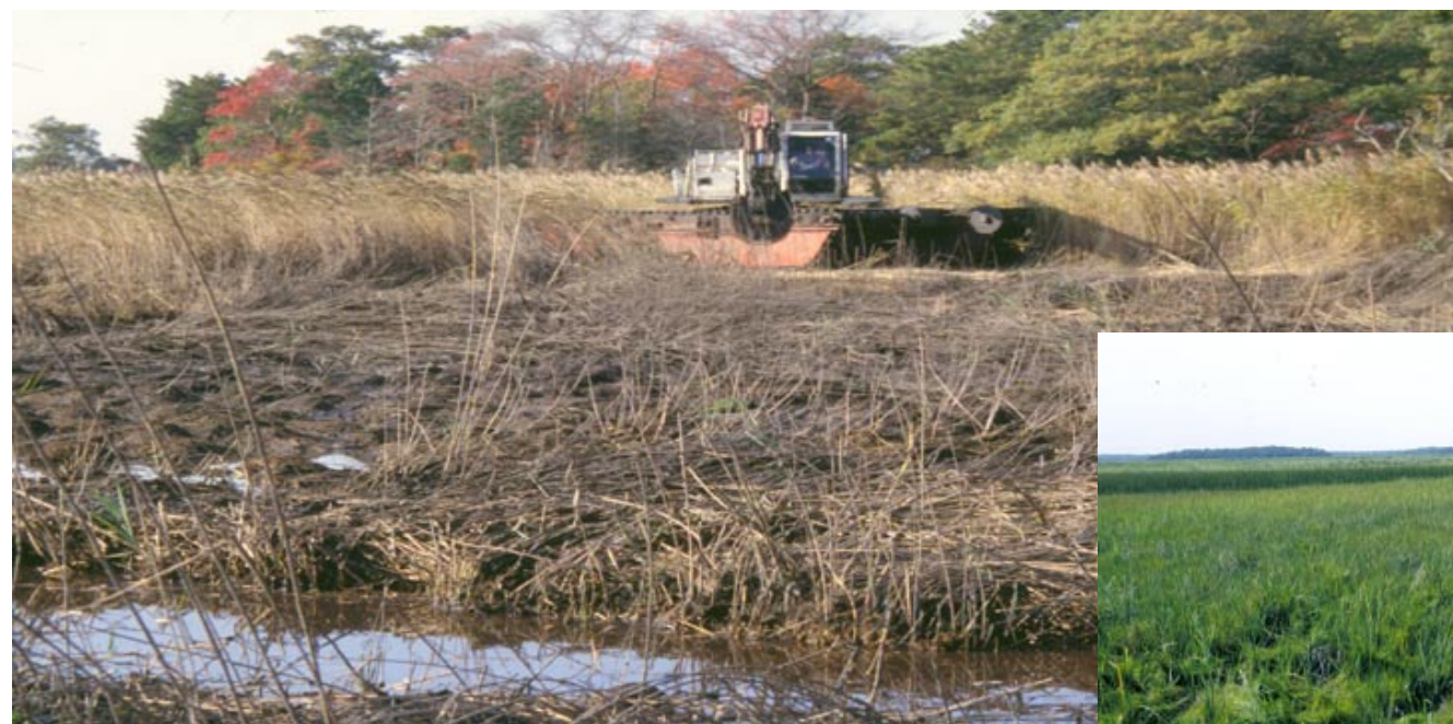
Digging tidal ditches to restore wetland hydrology along the New Jersey coast
