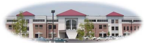
The completed MCVI in Saginaw, Michigan.
